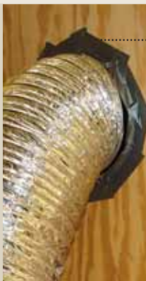
FIGURE 5 Window adapter with flex duct attached.
