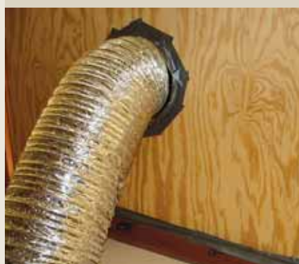
FIGURE 6 Flex duct connected to window template. The other end of the flex duct should be connected to the HEPA machine.
