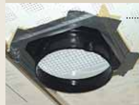
FIGURE 9 A return grille adapter.
