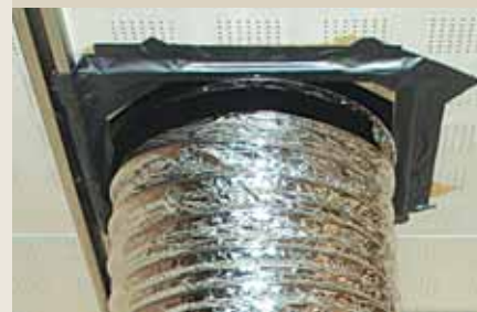
FIGURE 10 A return grille adapter with flex duct attached.
